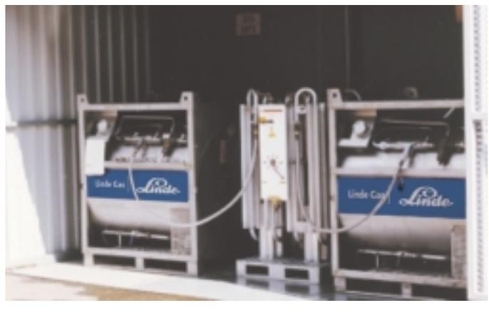
LIN tanks operate on the same principles regardless of the size or amount of LIN they store. The vessel has two walls, the inner shell made from stainless steel to accommodate the cryogenic temperatures and the outer shell constructed of structural steel. The space between the two walls contains an insulating material.
